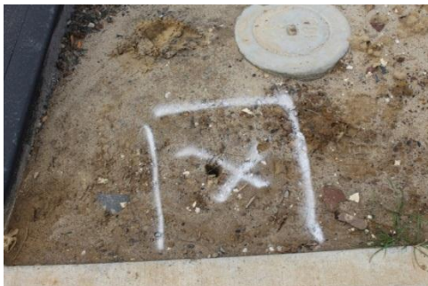
Use a spray can to mark the ground
