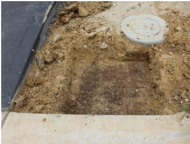
Dig the area out to the approximate dimensions and 100mm deep
